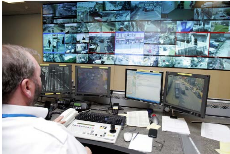
Fig. 1 –Control room screens
